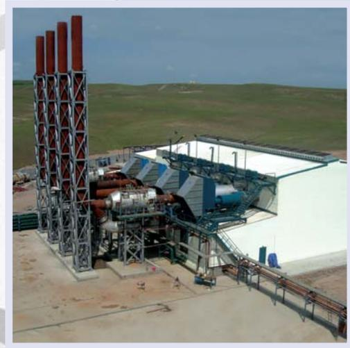
Erbil Steel Company produces the electricity required by its facilities via five 6.4 MW Wartsila diesel-generator groups, totaling 32 MW.
